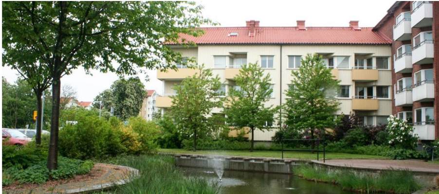
Fig. 3 The Sustainable Urban Drainage System developed through the initiative (World Habitat Awards 2010)
